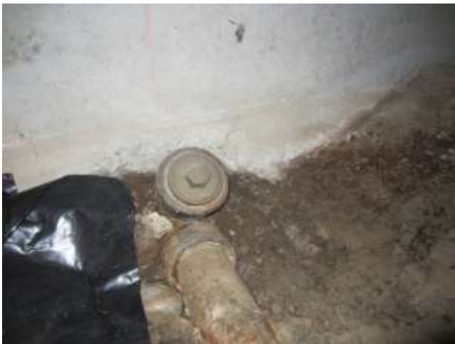
Cast iron waste line outfall near crawl access
