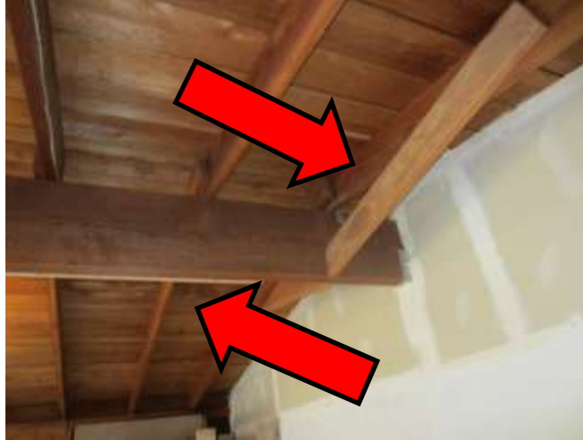
Rafter supports added 2 x scabbled onto side of beam
