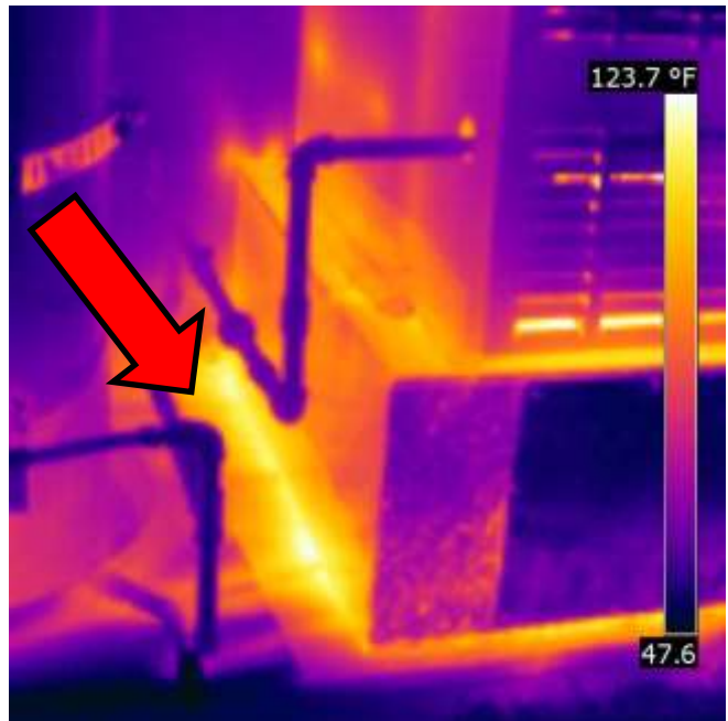
Air leakage at furnace
