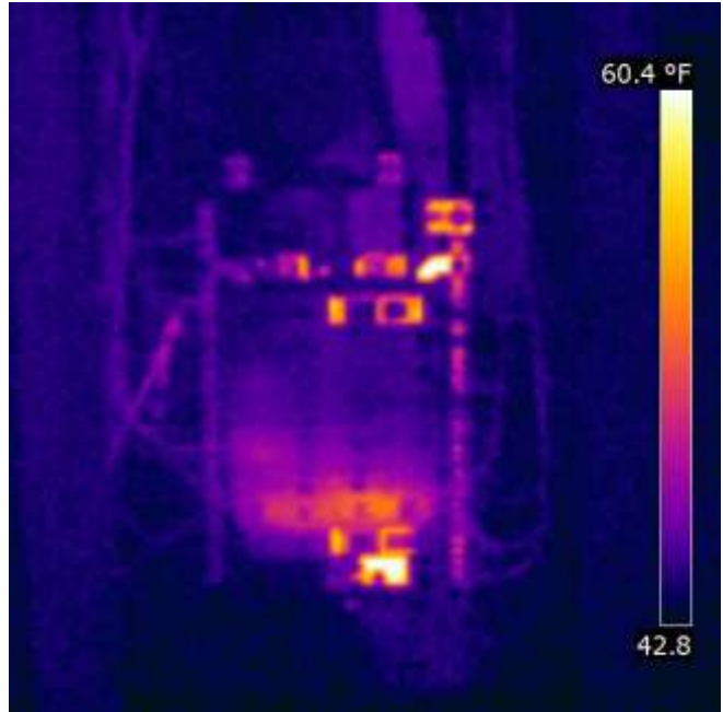
No evidence of over heating
