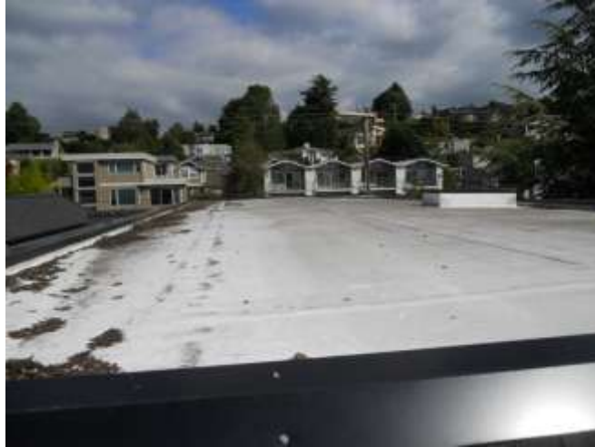
Membrane roofing Scuppers need to be clear of debris
