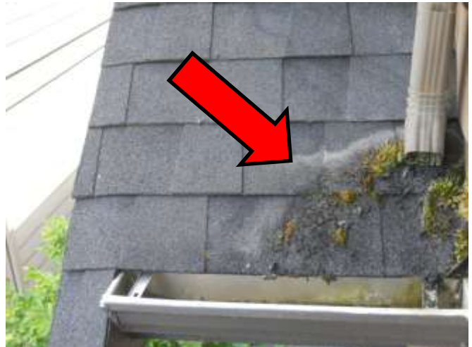
Gutter above and left of garage
