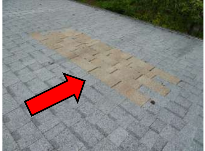
Roof repair at Kitchen
