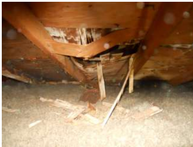
Sheathing at garage has (2) layers Lower sheathing has a hole cut in
