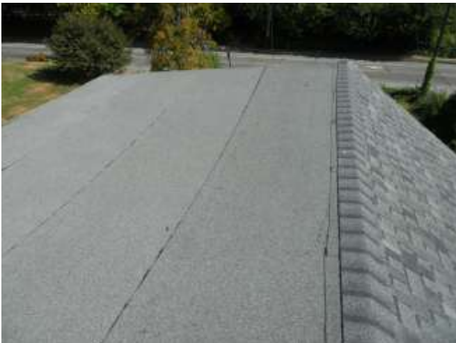
Upper roof area (facing East)
