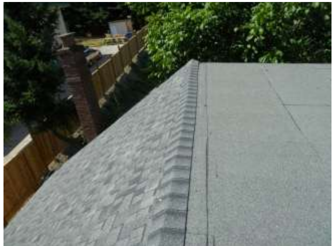
Upper roof area (facing West)
