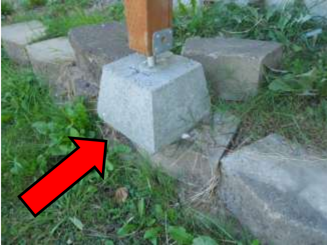
Pier pad placed on retaining wall block
