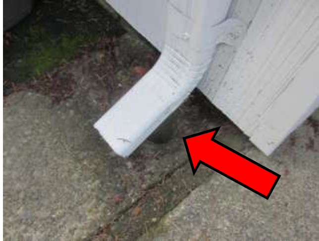
Downspout is directed away from underground drainage system
