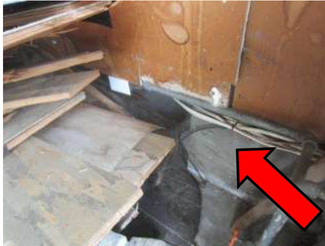
Possible access to below front porch
