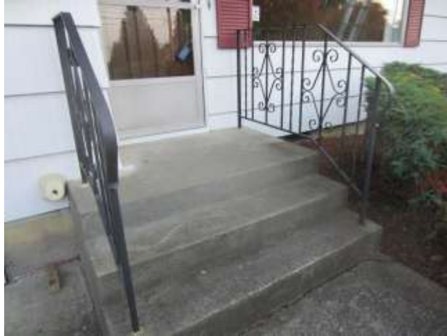
Appropriate handrail at front steps
