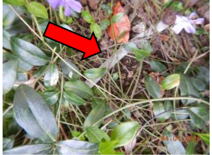
Unprotected wire in a planter bed
