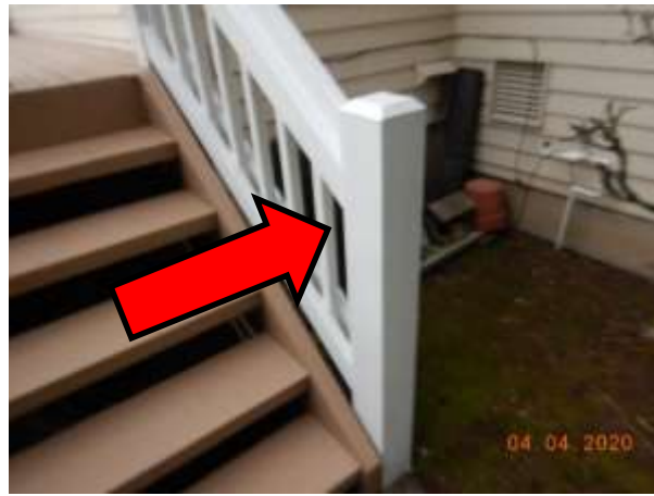
Loose handrail
