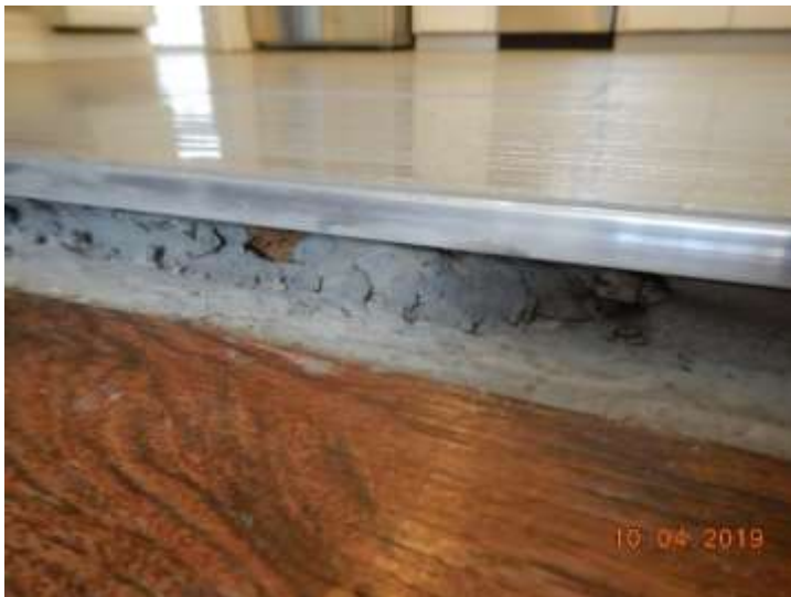
Large vertical height difference @ kitchen
