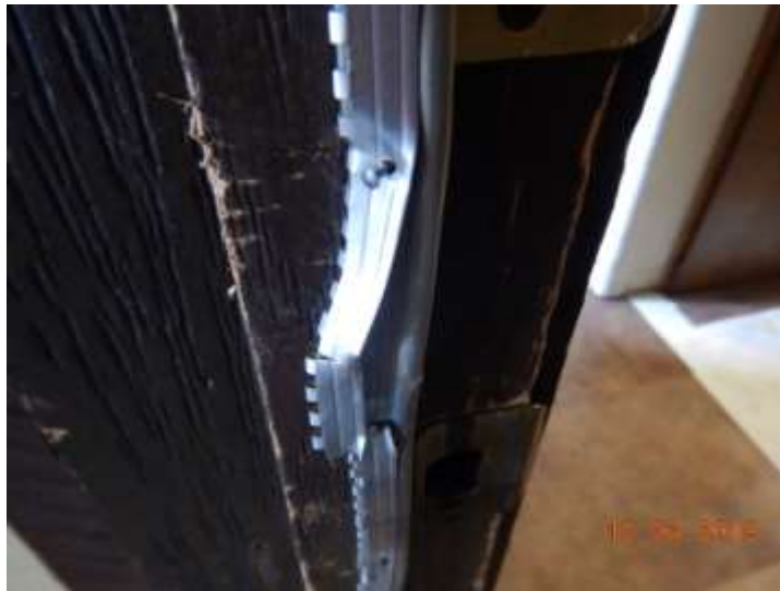
Damaged weather-stripping
