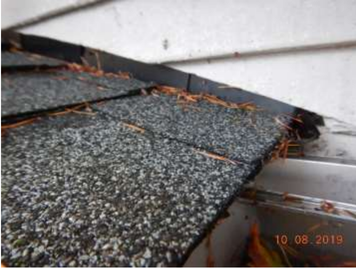
Proper diverter flashing is installed
