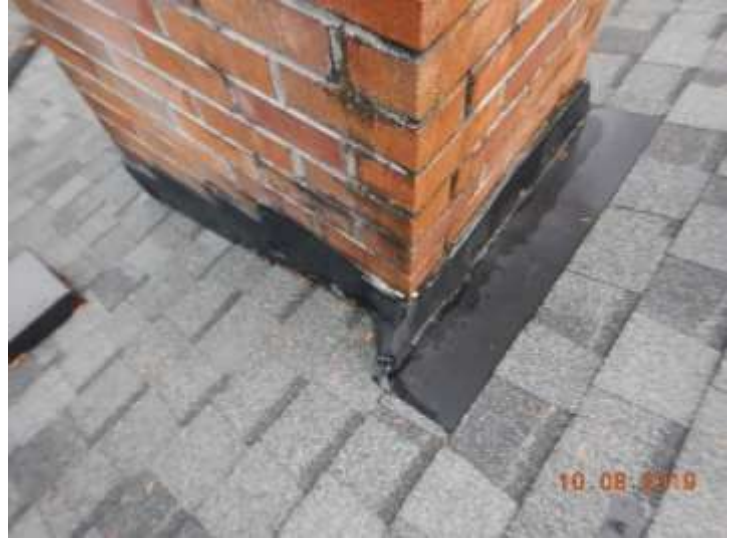
Chimney flashing
