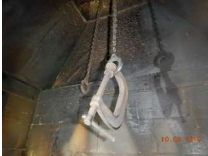
The damper is held in place by a c clip
