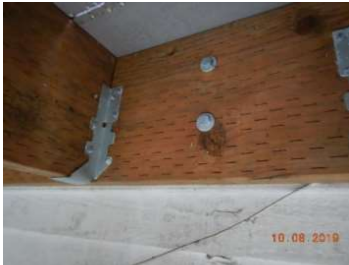
The deck is properly lag bolted to the home
