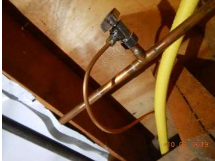
The water supply to the refrigerator appears to be located in the workspace below
