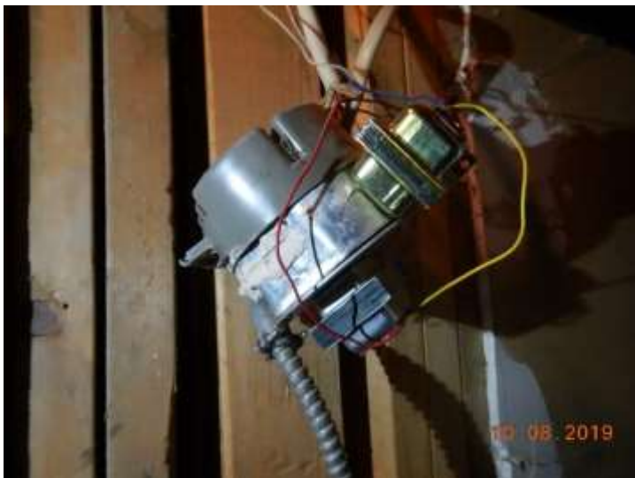
Unsecured wiring
