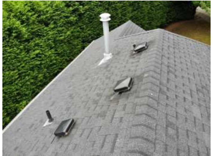
Furnace flue
