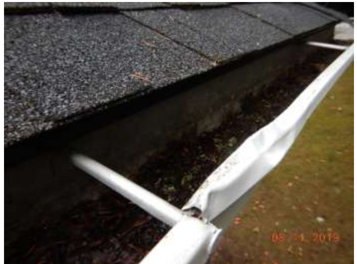
Dented gutter
