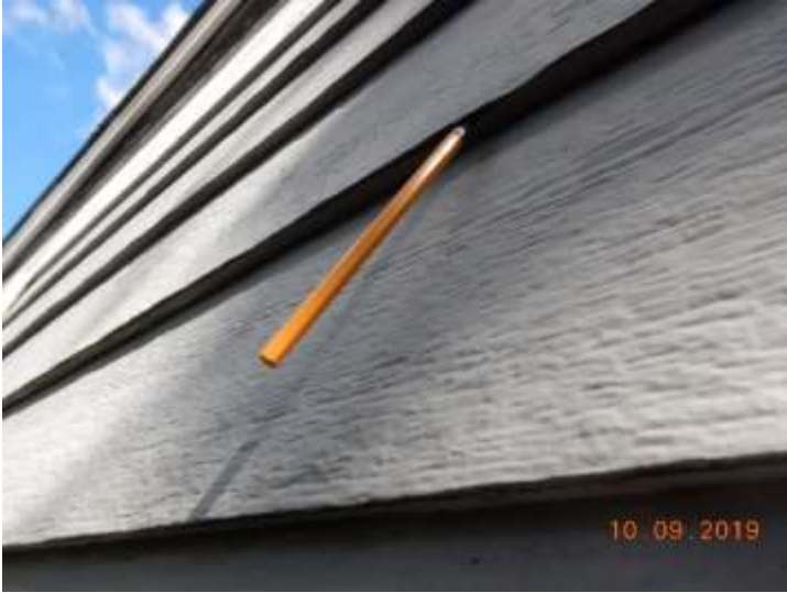
A probe can be easily pushed into the lower edge of the siding
