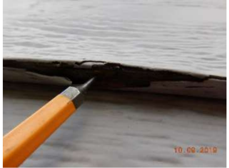
Probe pushed into the siding
