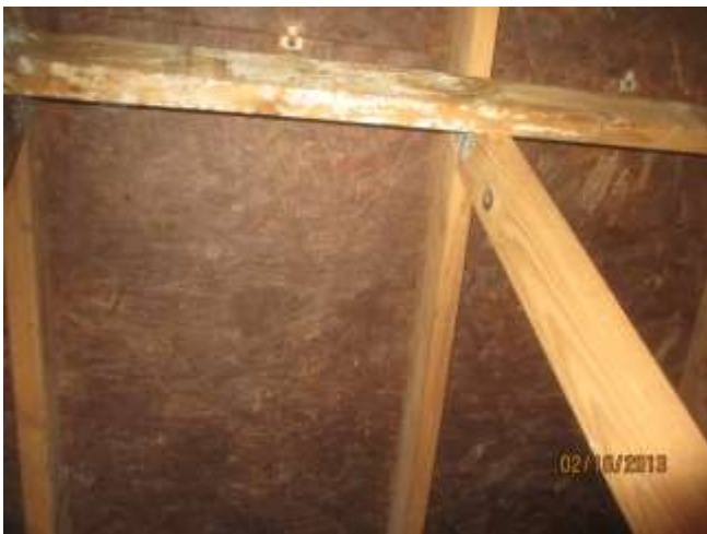
Evidence of microbial growth
