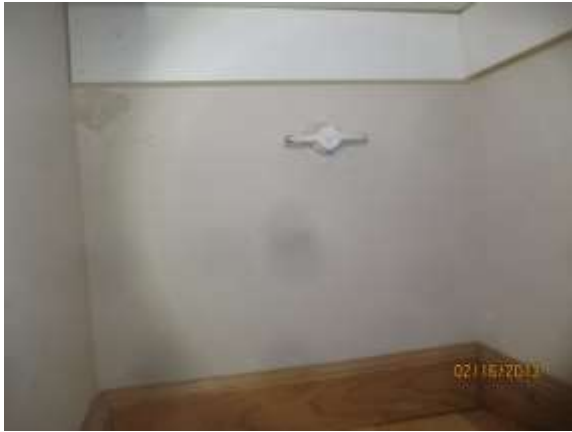
Domestic Water Shut off
