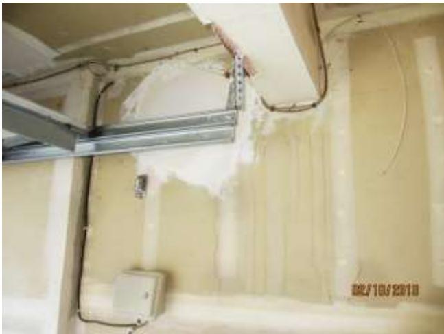
Moisture stains at the South wall and beam
