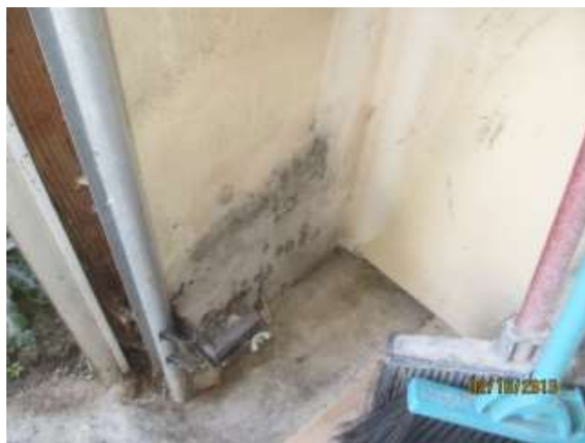
Moisture stains at the South wall and beam
