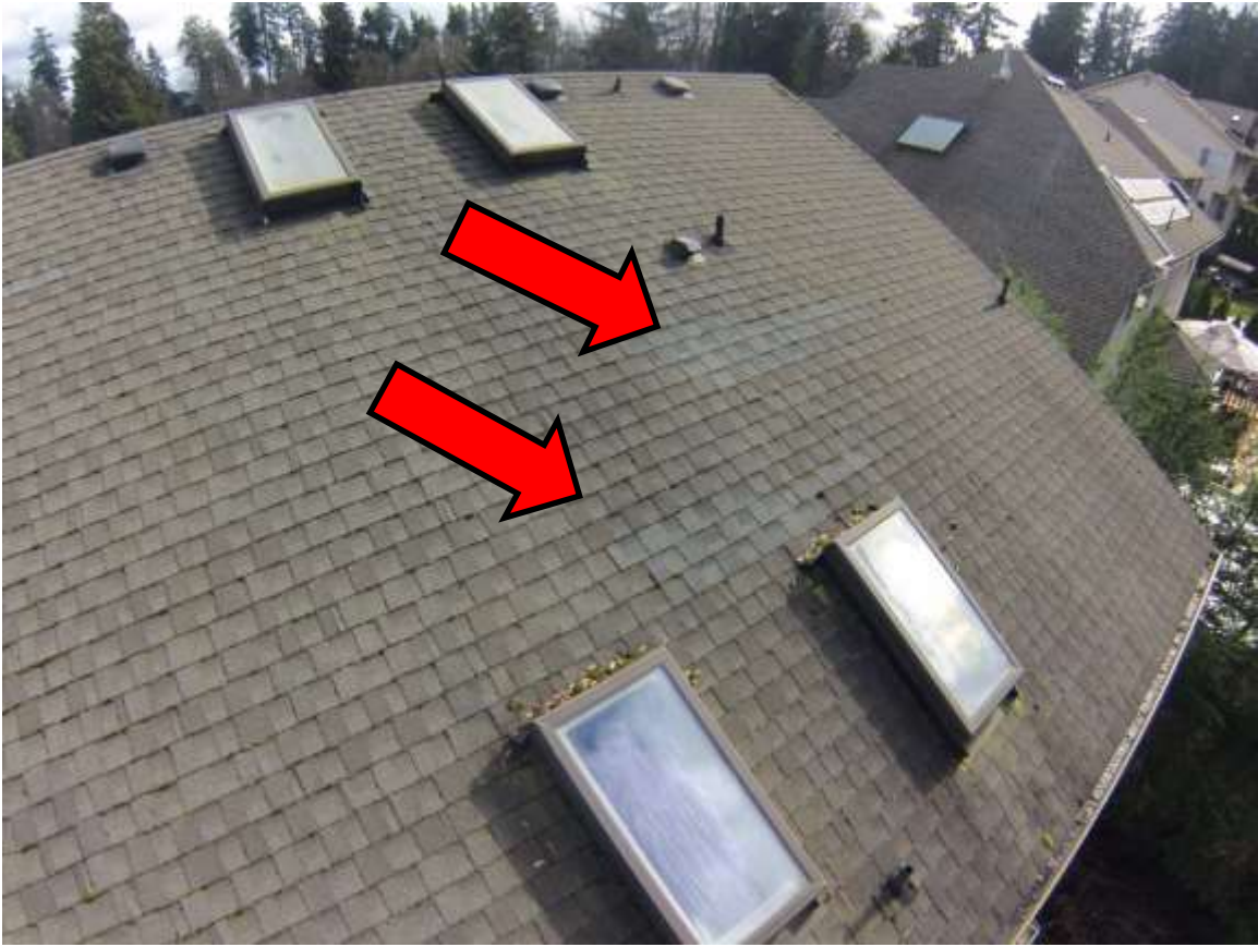
Roof repairs above the Master bathroom area
