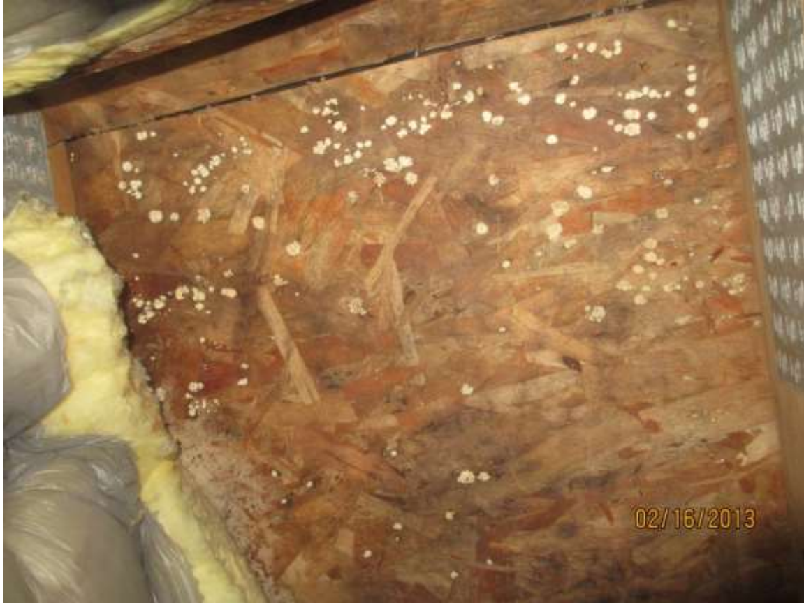
Evidence of microbial growth
