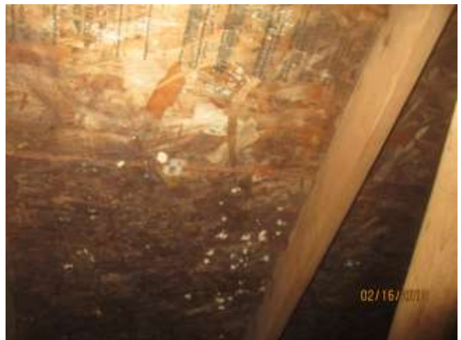
Evidence of microbial growth
