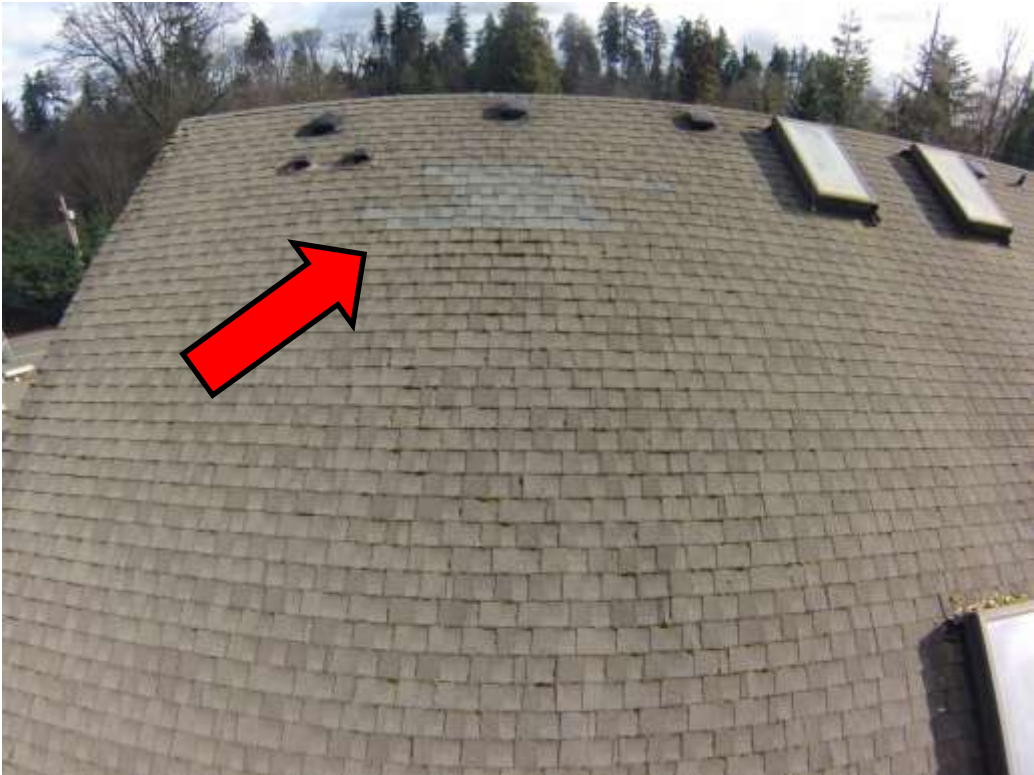
Rear roof repair at the Master bedroom area
