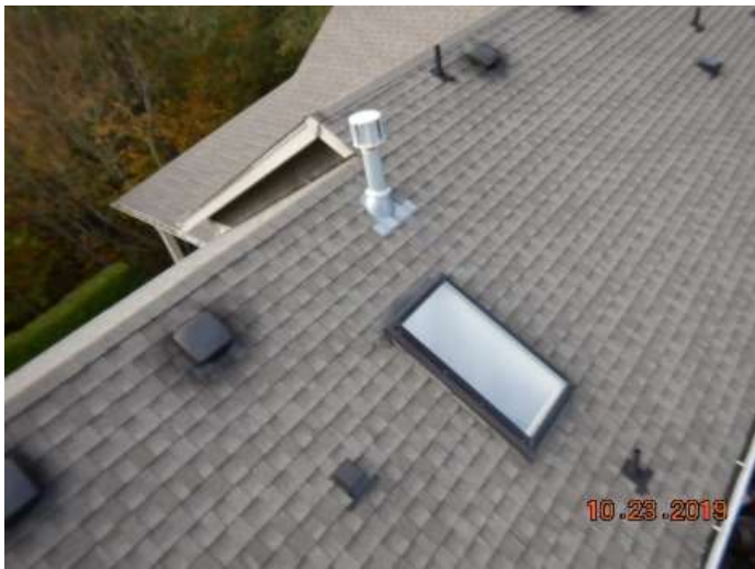
Furnace flue and skylight
