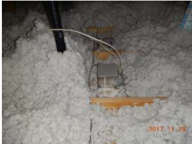
Missing insulation
