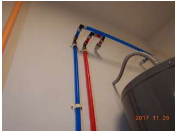
Missing pipe insulation
