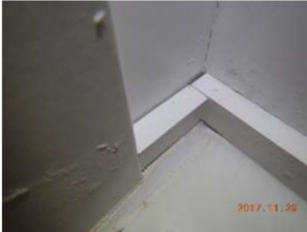
The material used for base shoe is not a ¼ round as used throughout the industry. Corners are blunt cut and not caulked
