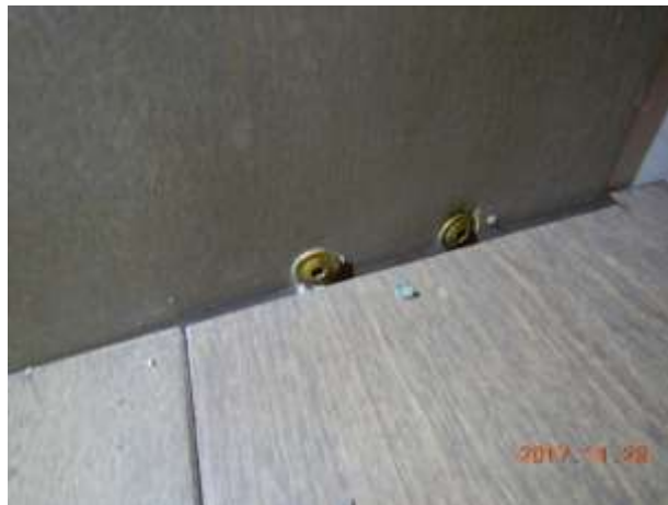
Screws visible at the stairwell barricade post. It may be possible that the builder was planning to add base shoe to this area
