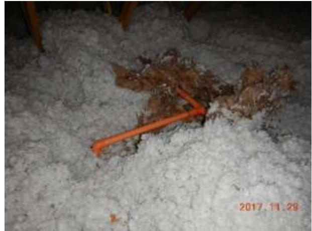
Exposed fire suppression system pipes
