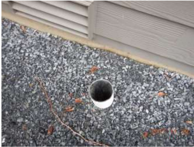
Open drain pipe
