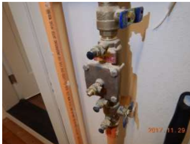
The fire suppression valves are in the off position
