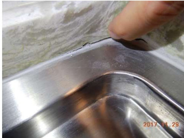
Large gaps at the corners of the sink
