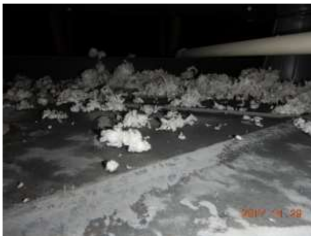
Debris in the drip pan
