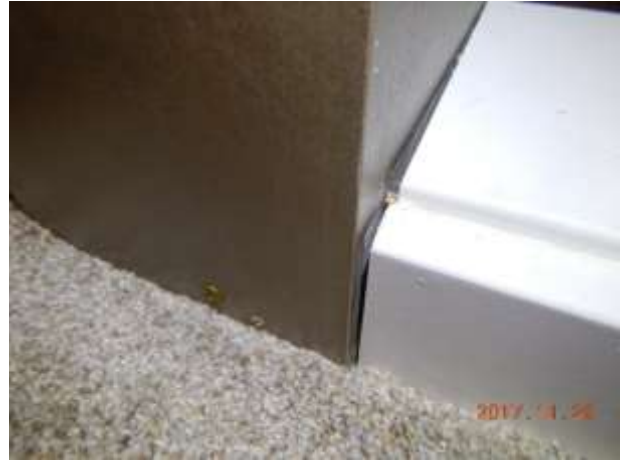
Large gaps adjacent to the stairwell barricade post
