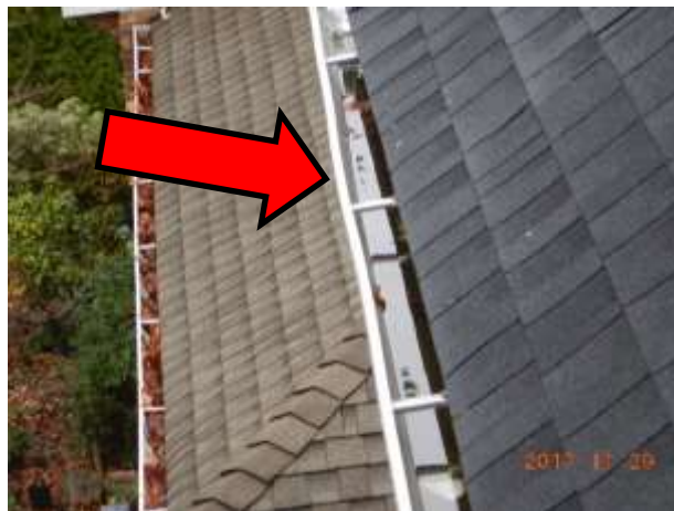
Standing water in the gutters
