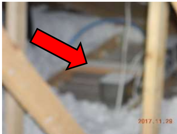
Missing insulation
