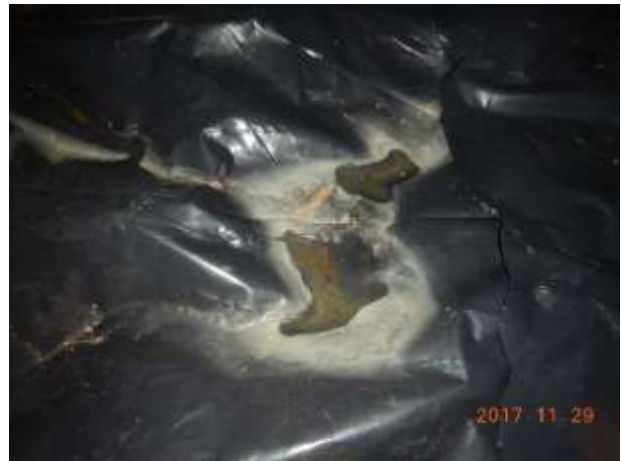
Puddles of water on top of the vapor barrier
