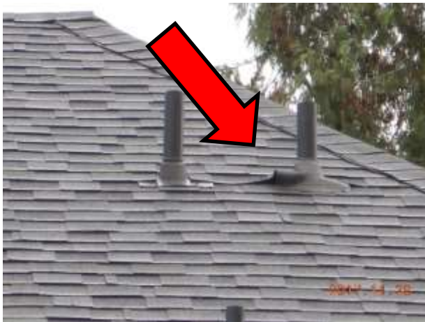
Raised side of a plumbing vent
