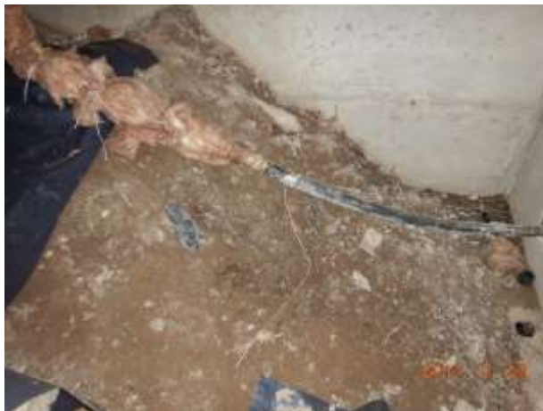
Missing vapor barrier
