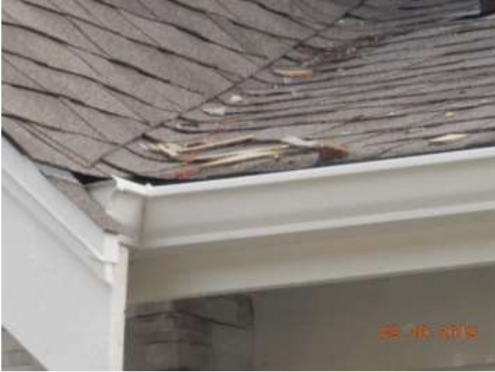
Debris on the lower roof
