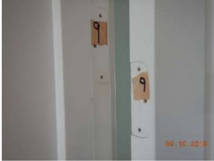
Hinge locations do not line up
