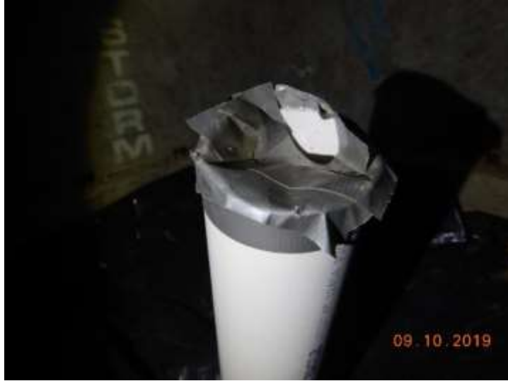
The crawlspace drain pipe should be tightly screened to prevent rodent intrusion
