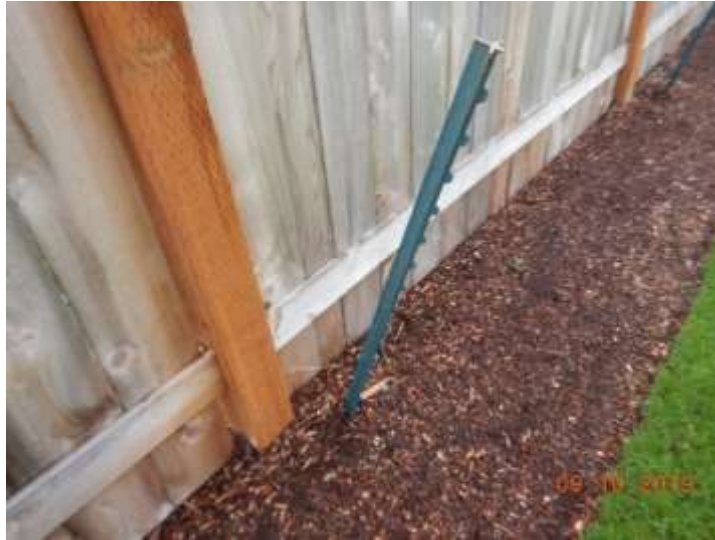
Metal posts at the rear yard
