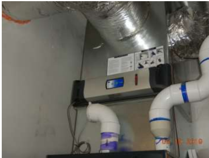
Furnace filter location
