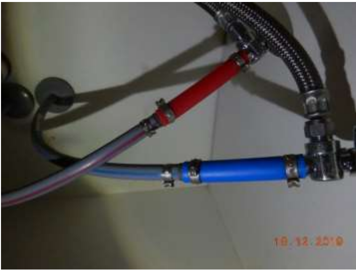
Pex pipe was spliced onto the piping to the sinks
