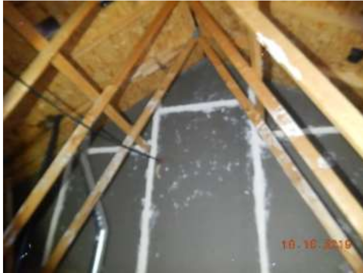
A unit to unit firewall is installed
