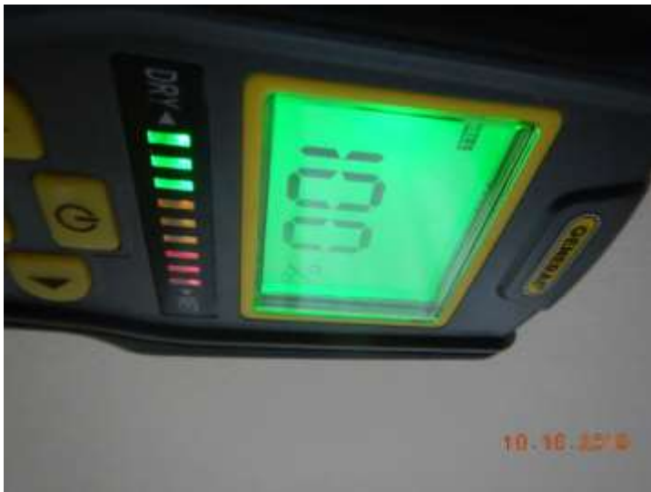
High moisture reading
