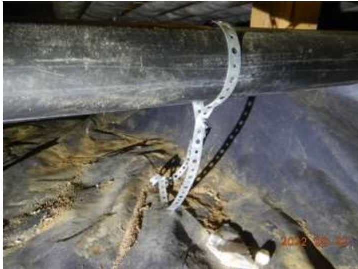
Disconnected support band
