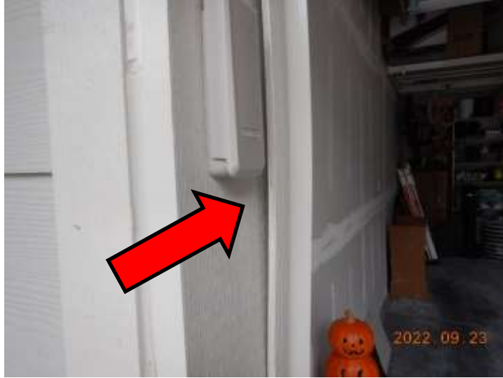
Loose weatherstripping
