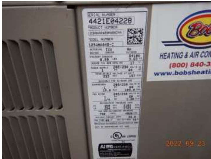
A/C system compressor information tag
