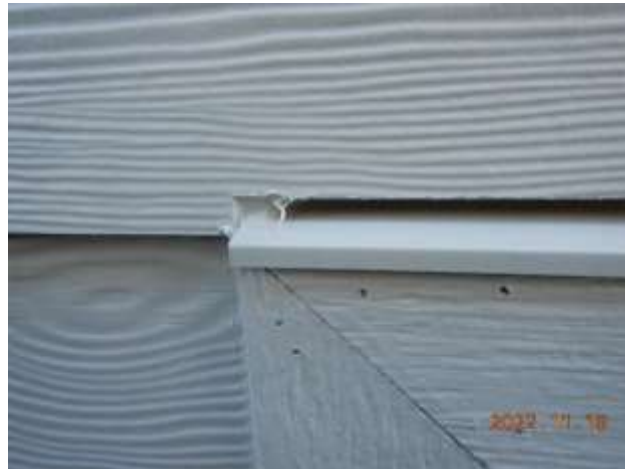
Proper head flashings are installed
