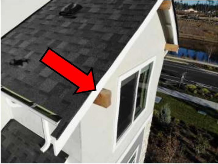
Exposed false beam
