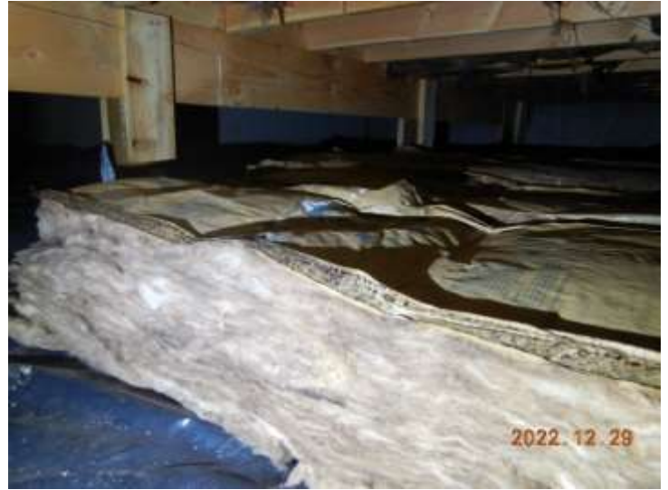
Insulation laying on the vapor barrier
