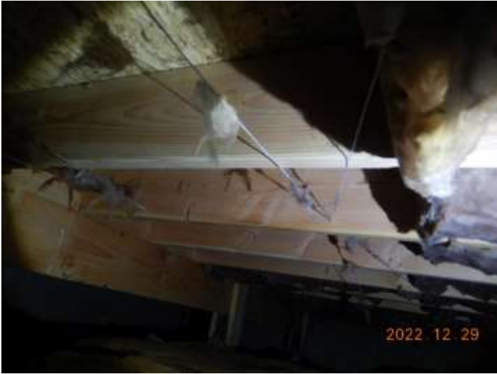
Missing insulation
