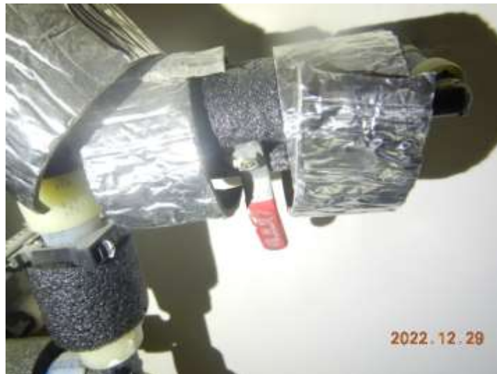
The hose bib located at the garage area is turned off (winterized); not tested.
