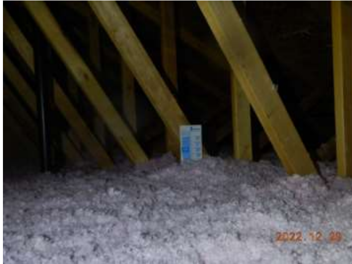
Insulation depth measurement in the Attic (measurement by others)
