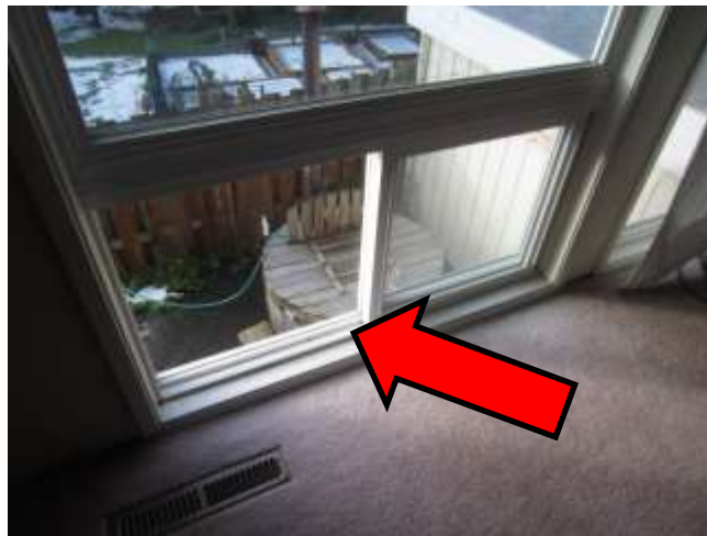
Windows open at floor height
