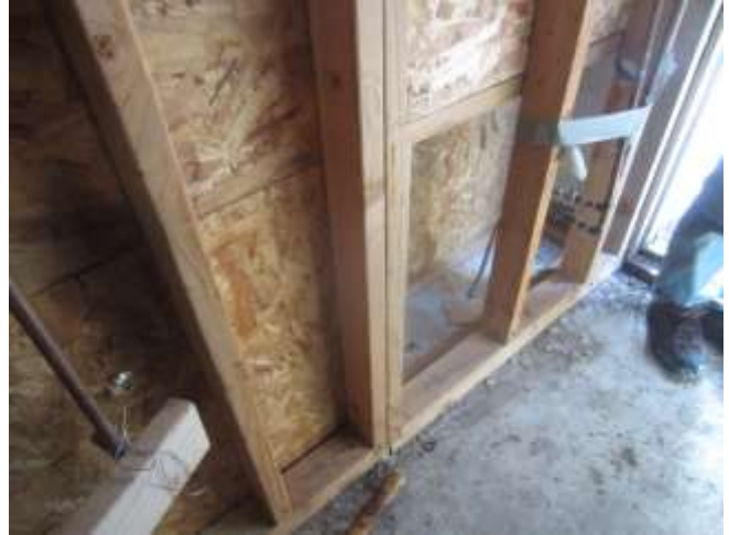
Partition separating the new bathroom and remaining storage shed area
