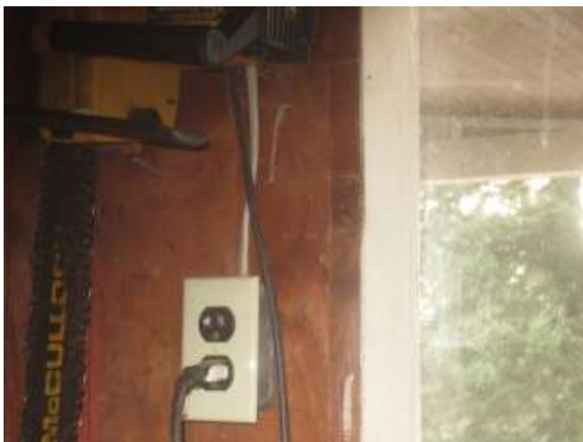
New electrical outlet
