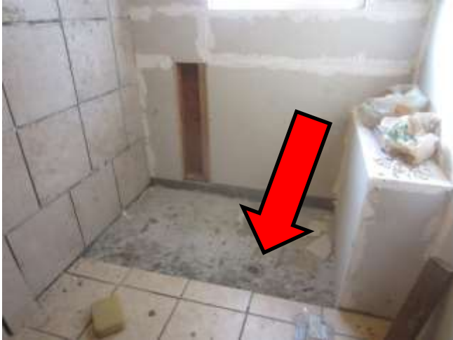
Waste line is covered by concrete floor
