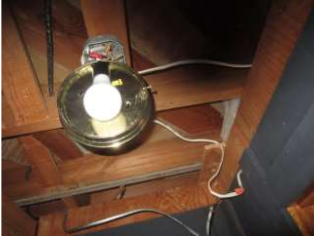
Light fixture hanging in storage room
