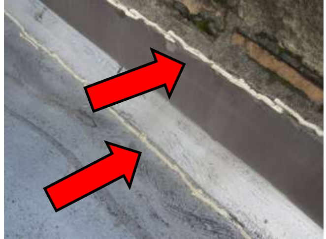
Caulking repair at chimney flashing
