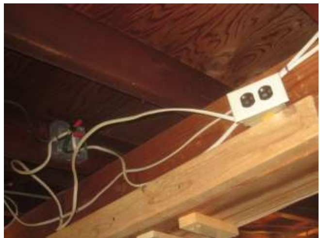
New wiring in the garage
